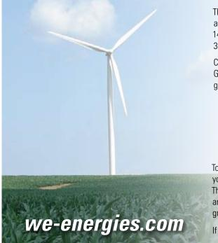
The Blue Sky Green Field Wind Energy Center, located in the towns of Calumet and Marshfield in northeast Fond du Lac County, is designed to generate 145 megawatts (MW) of electricity, and is capable of powering approximately 36,000 average residential homes. The site consists of 88 wind turbines.
